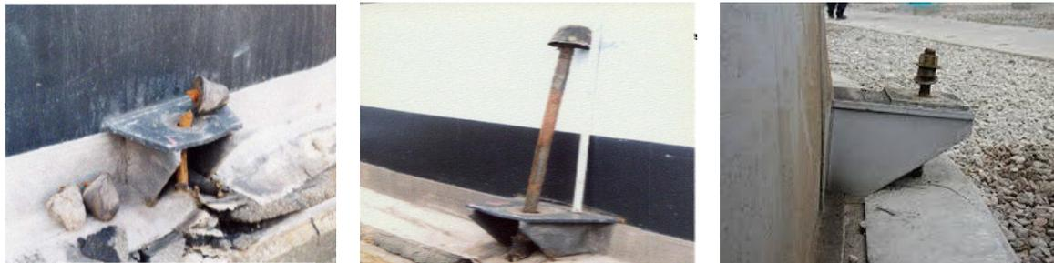
Fig 6: Tank anchored bolts have been cut or coming out by the earthquake
