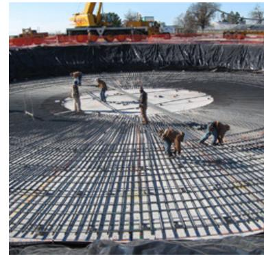
Fig. 4: Foundation of cylindrical steel tanks
