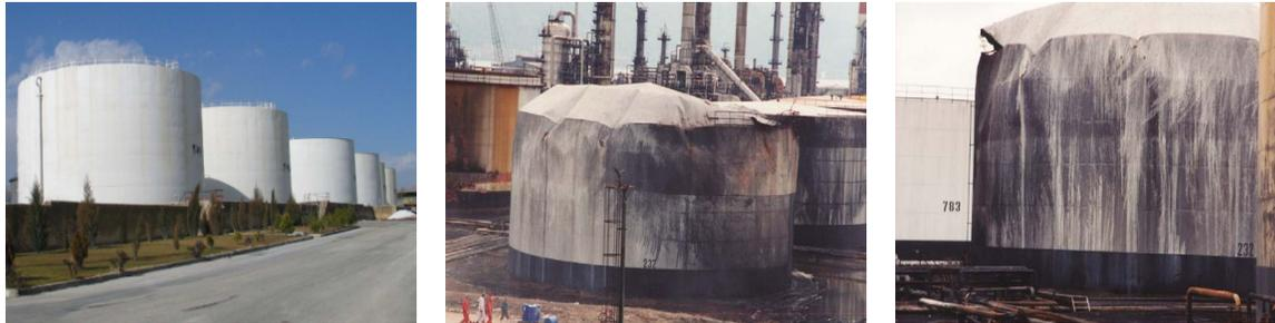
Fig. 1: Steel storage tanks and tanks damaged by the earthquake
