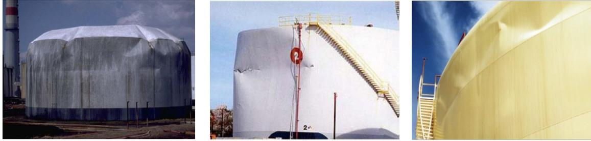
Fig. 5: The roof and upper part of the tank shell damaging caused by sloshing phenomenon
