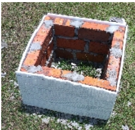
Fig. 2: Clay brick wall that apply polystyrene before plastering
